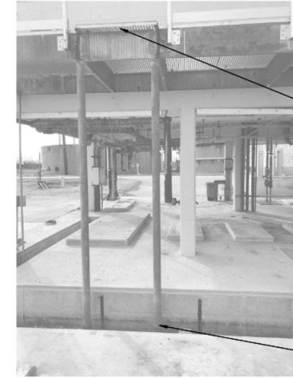
STORM SHELTER UPPER WALKWAY COLUMN REPAIR SCALE: NONE
